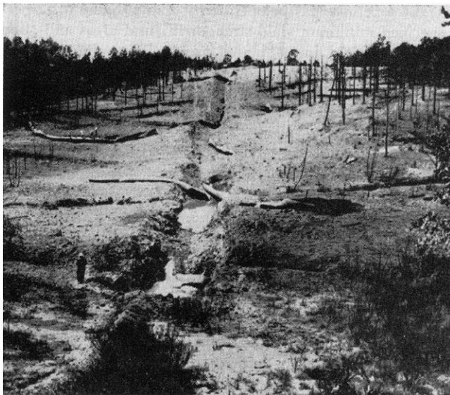
Figure 5.28. Pipeline that failed during testing. From E. R. Parker, Brittle Behavior of Engineering Structures , John Wiley and Sons, 1957.
